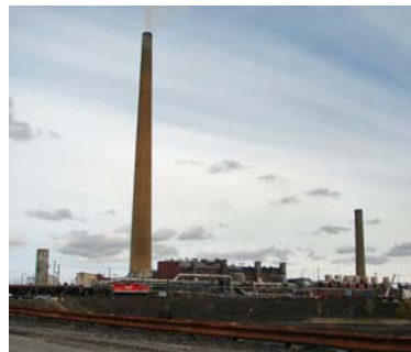
Inco's 1234 ft Superstack
